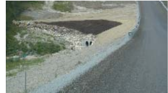
Culvert and dissipator adjacent to the mine access road
