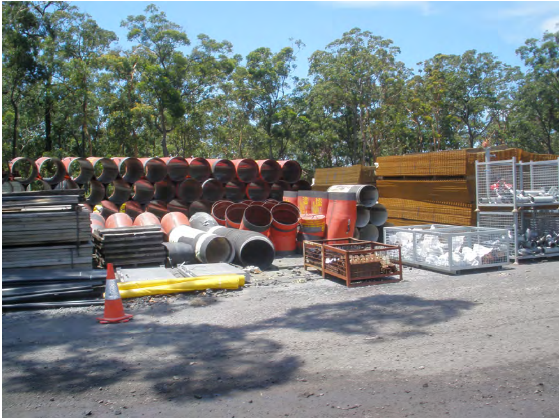
Plate 7 - Laydown area for materials
