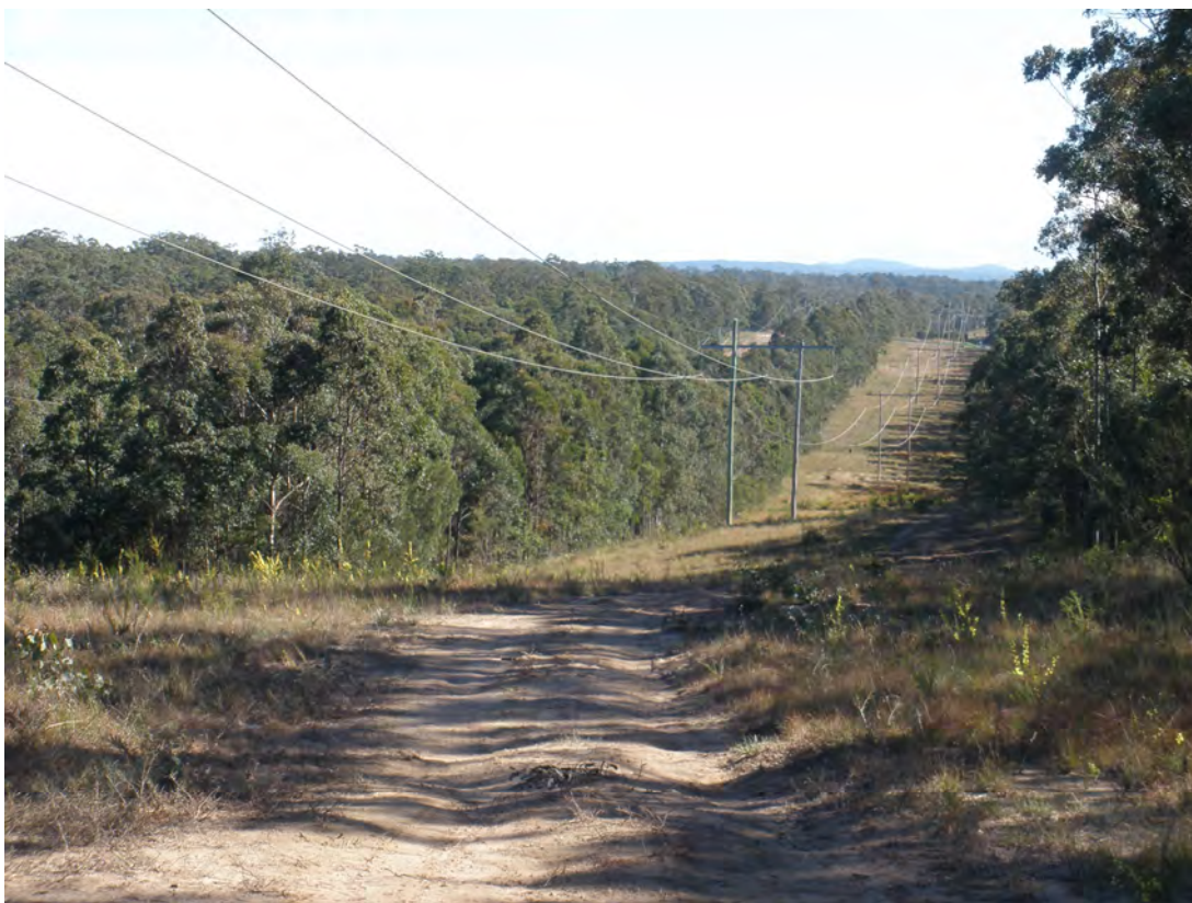
Figure 6 - High Voltage Transmission Line Easement on the Site
