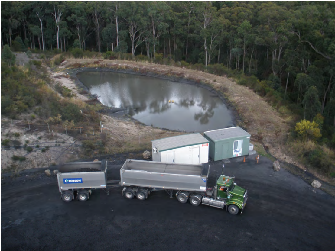
Plate 6 – Pollution control dam and haul truck
