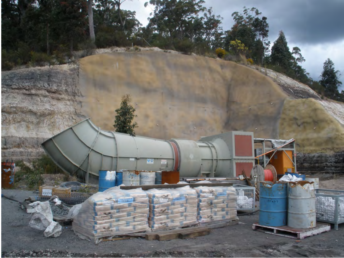
Plate 3 - Laydown area and ventilation adit
