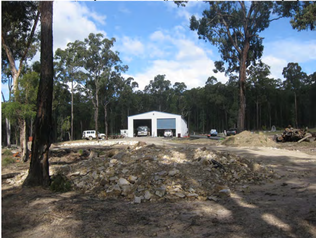
Commercial workshop / office building (Lot 9) in western area of proposed mine site
