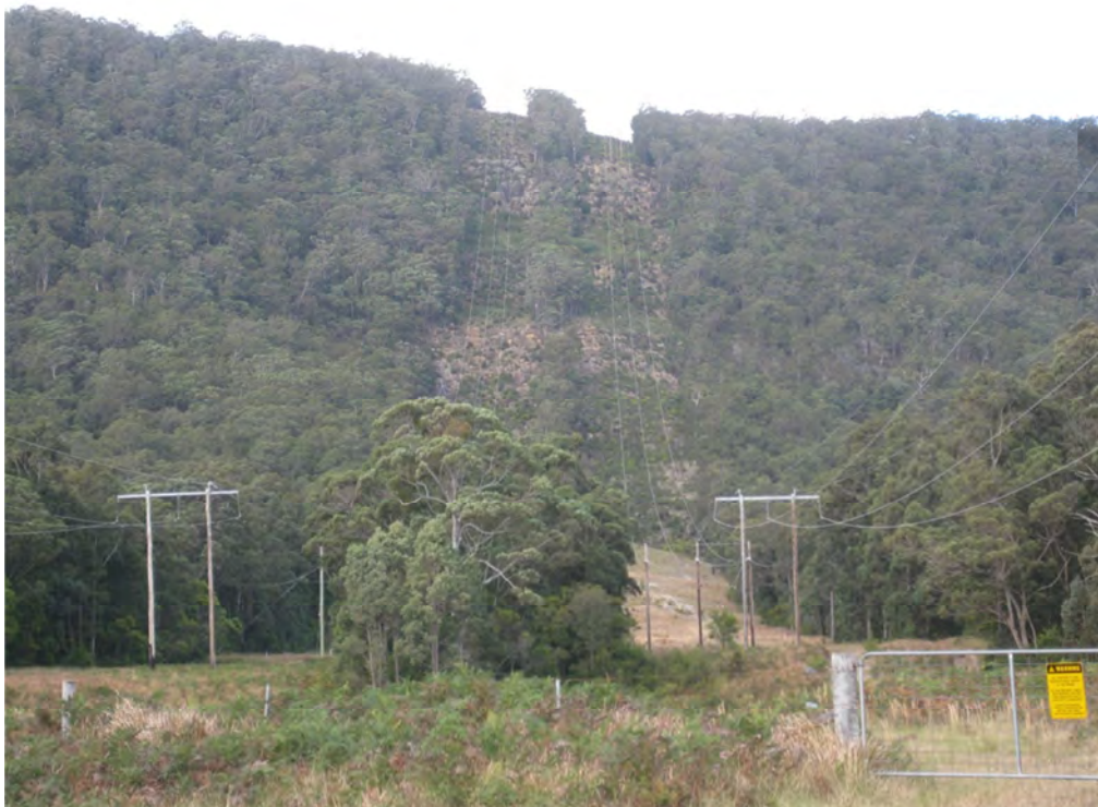
Ausgrid 132kV & Telstra FOC (along RHS) easement and west facing ridge crest & steep slopes in south eastern area of proposed mine site
