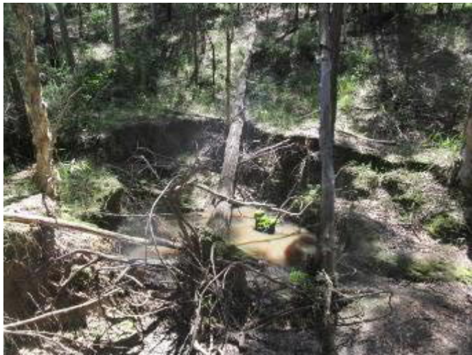
Plate 85 – Erosion Downslope of Sediment Dam E
