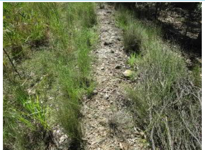
Plate 72 – Contour Bank Upslope of Sediment Dam D
