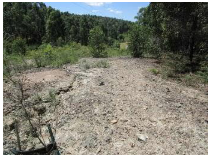
Plate 94 – Eroded Channel Upslope of Rumbles Dam
