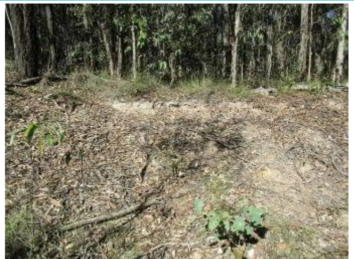
Plate 18 – Sediment Dam B Spillway
