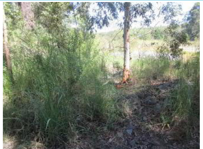
Plate 60 – Sediment Dam D Spillway
