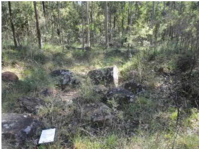
Plate 13 – Sediment Dam A Spillway
