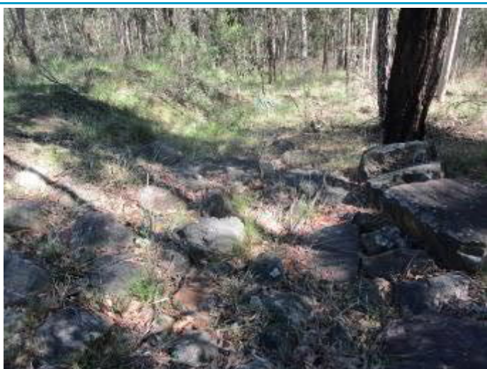
Plate 29 – Sediment Dam C Spillway
