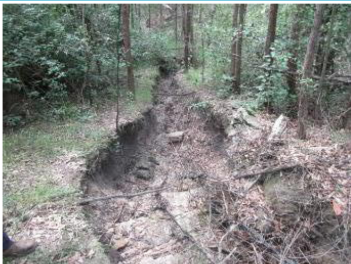
Plate 106 – Erosion Downslope of Rumbles Dam
