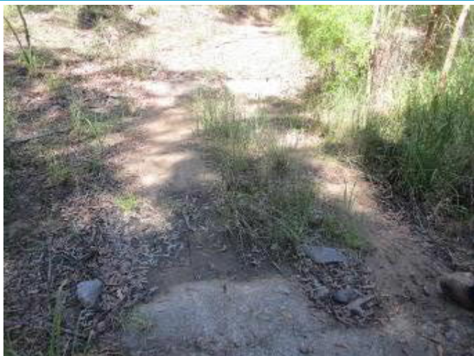
Plate 59 – Sediment Dam D Spillway
