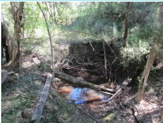
Plate 83 – Erosion Downslope of Sediment Dam E
