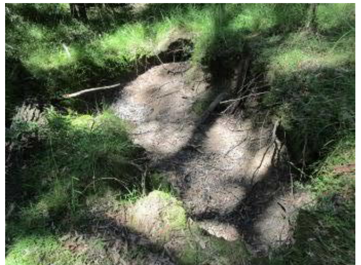
Plate 88 – Erosion Downslope of Sediment Dam E
