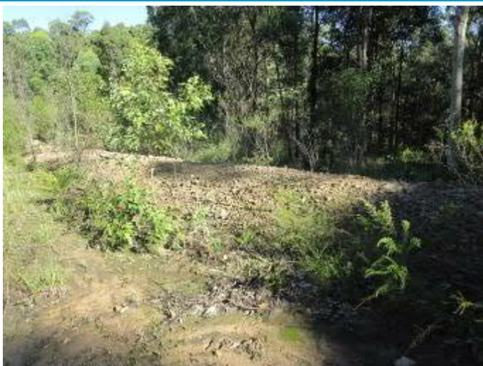
Plate 3 – Sediment Dam A Upslope Channel
