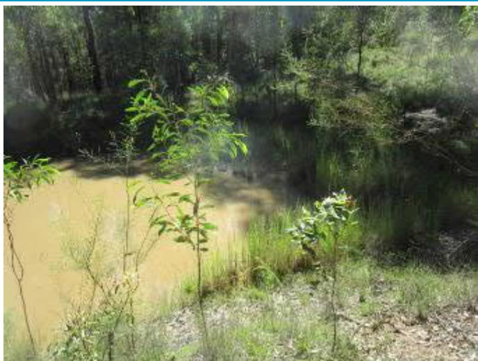
Plate 27 – Sediment Dam C
