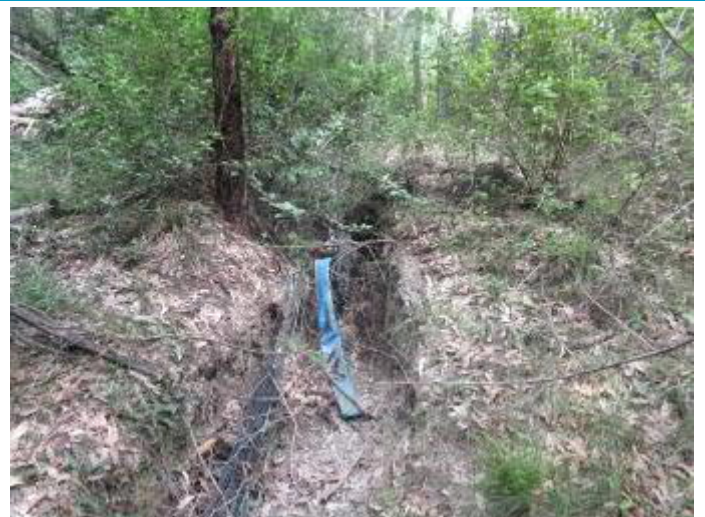
Plate 107 – Erosion Downslope of Rumbles Dam
