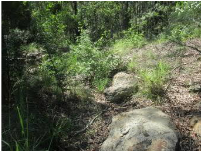
Plate 61 – Sediment Dam D Spillway
