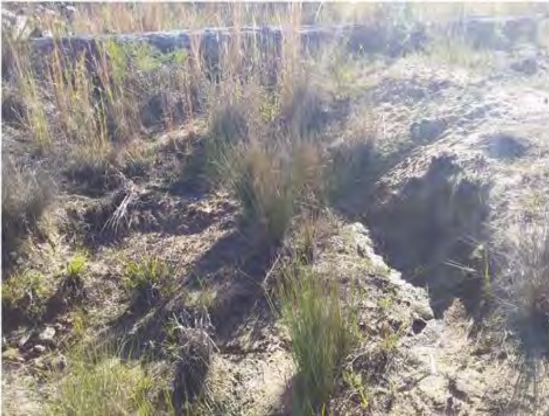
Photograph 3 Potentially Dispersive Soils in Banks of Sediment Dam 3 Storage
