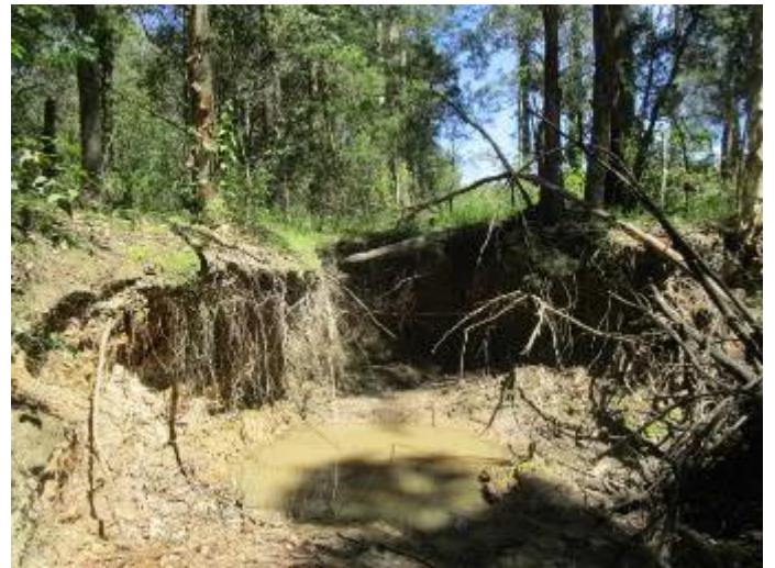
Plate 86 – Erosion Downslope of Sediment Dam E
