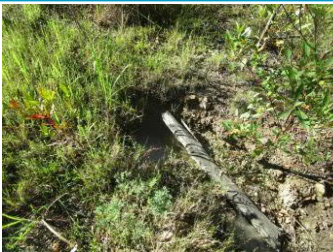
Plate 5 – Sediment Dam A Upslope Channel
