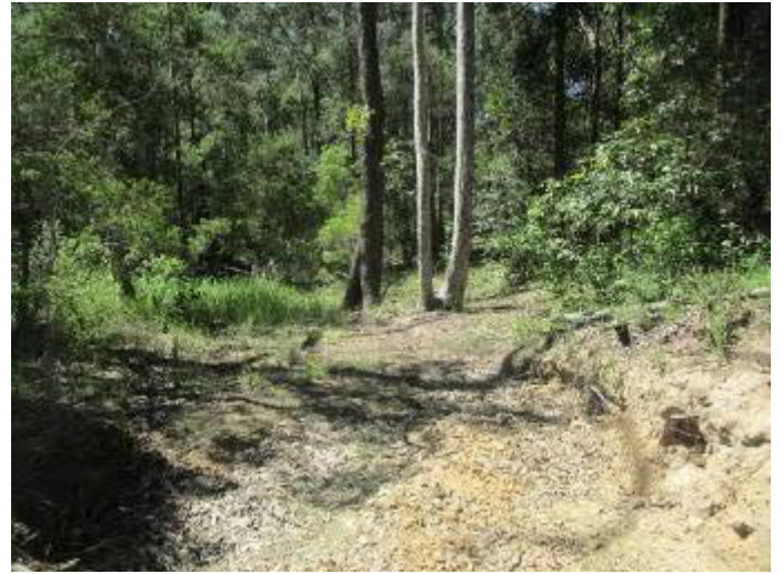
Plate 80 – Sediment Dam E Spillway
