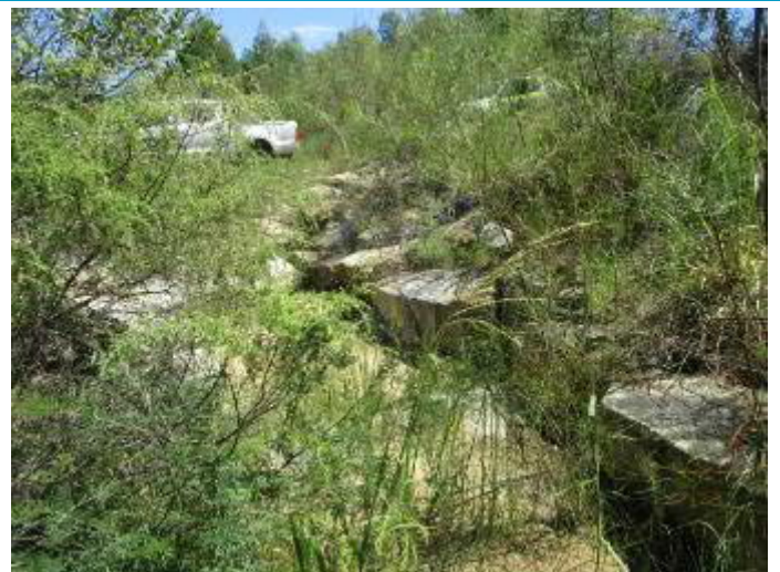
Plate 90 - Channel Upslope of Sediment Dam E
