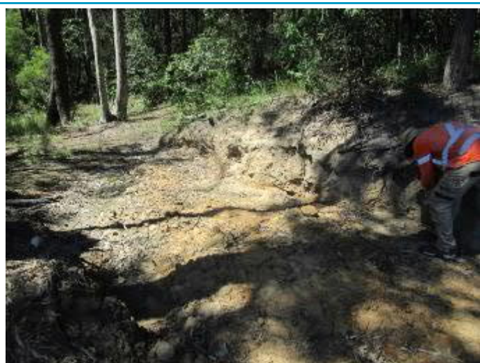
Plate 78 – Sediment Dam E Spillway
