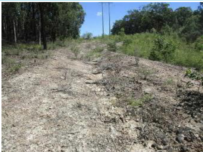
Plate 95 – Eroded Channel Upslope of Rumbles Dam
