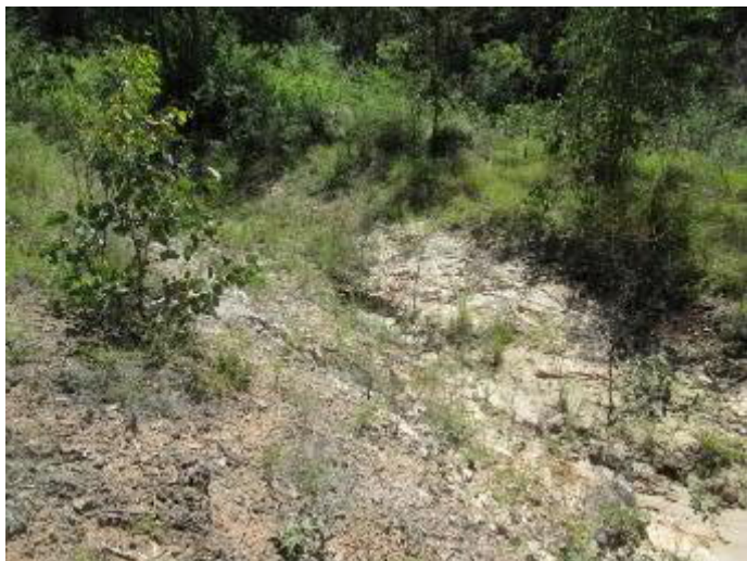
Plate 99 – Eroded Channel Upslope of Rumbles Dam
