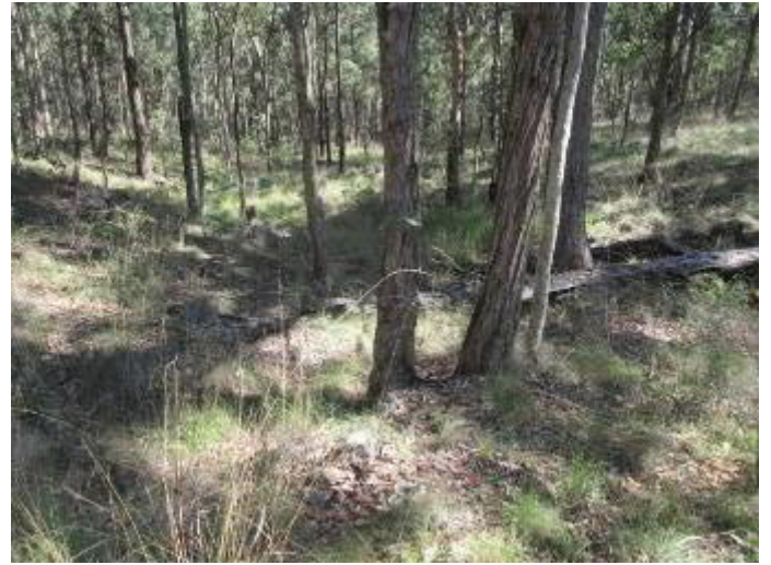
Plate 20 – Sediment Dam B Downslope of Spillway
