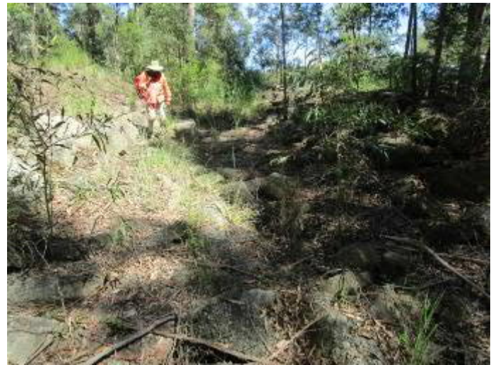
Plate 62 – Sediment Dam D Spillway
