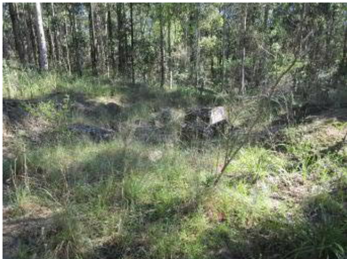
Plate 11 – Sediment Dam A Spillway
