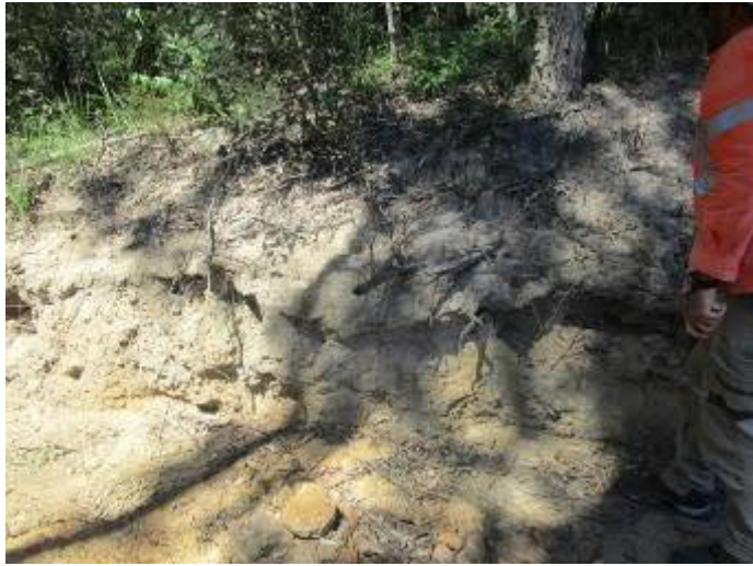
Plate 79 – Sediment Dam E Spillway
