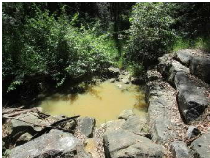
Plate 63 – Sediment Dam D Spillway
