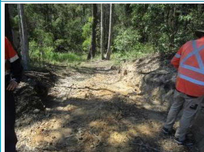
Plate 77 – Sediment Dam E Spillway
