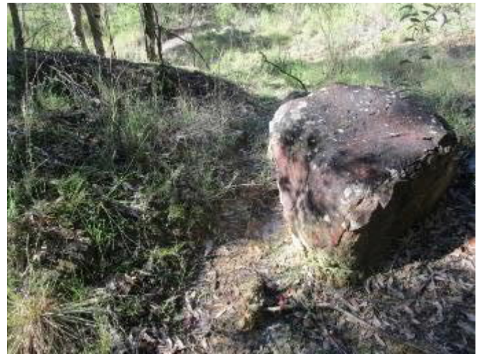
Plate 14 – Sediment Dam A Spillway
