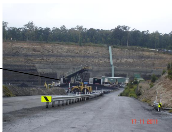
Abel Coal Mine portal with high wall and vegetation screening along John Renshaw Drive.
