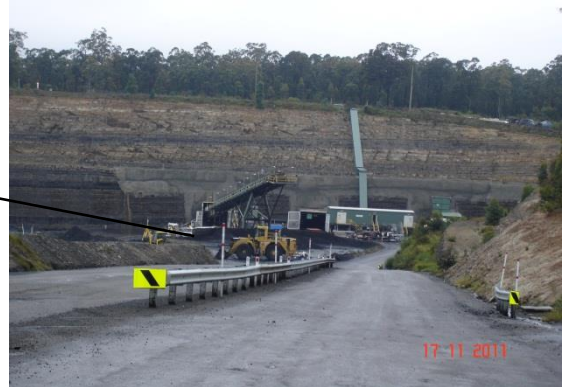
Abel Coal Mine portal with high wall and vegetation screening along John Renshaw Drive.
