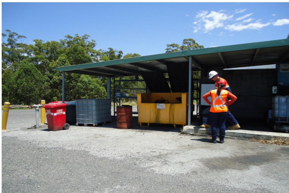
Plate 16 Well managed hydrocarbons storage area
