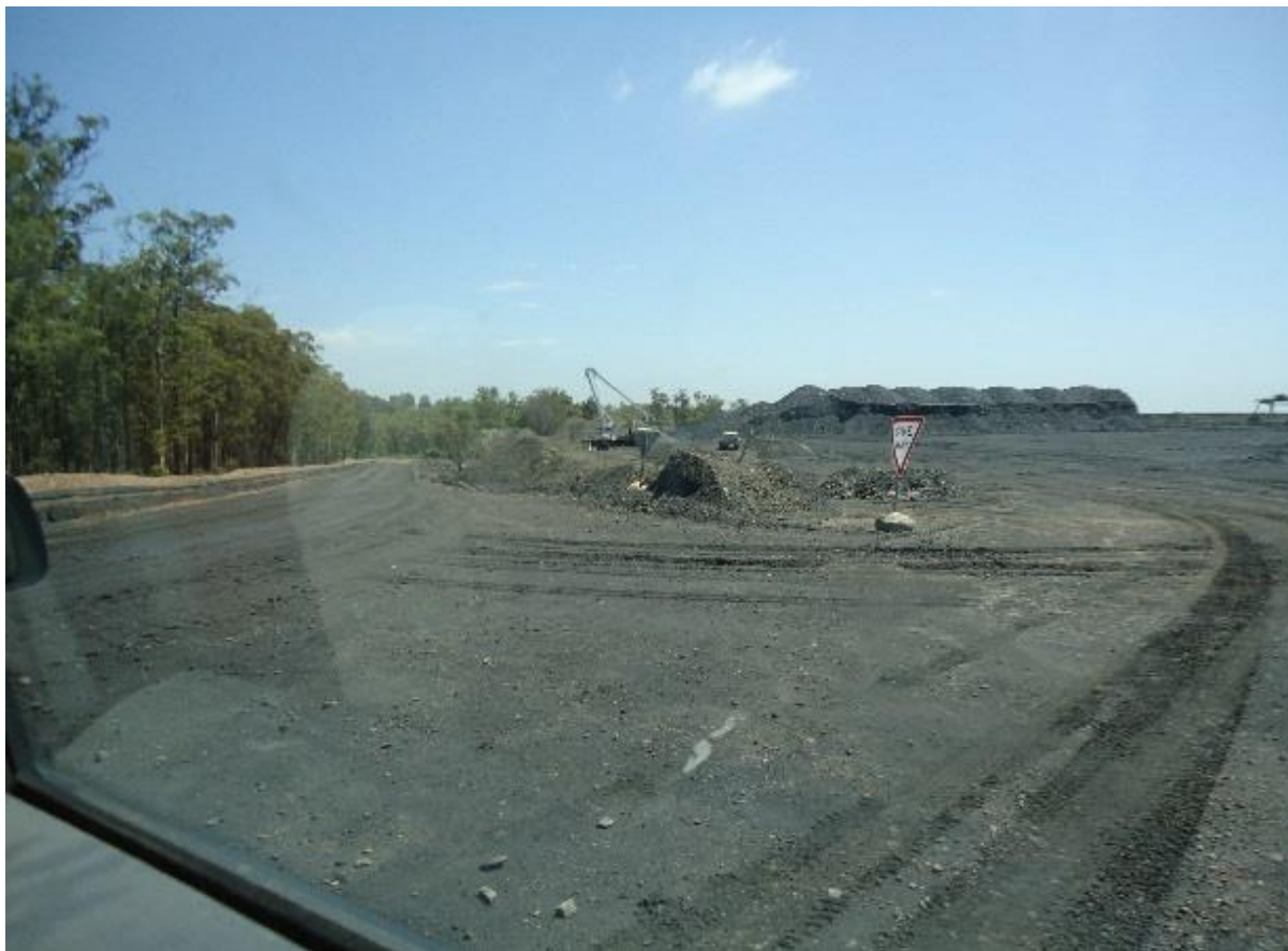
Plate 3 CHPP Bunding in place along Four Mile Creek
