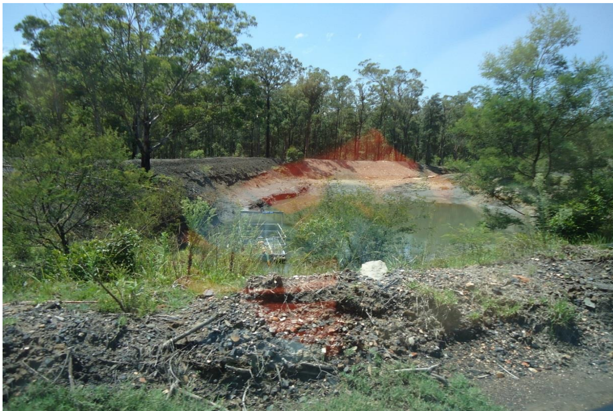
Plate 5 CHPP Sediment Dam recently desilted
