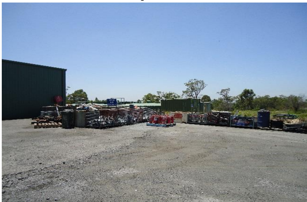
Plate 12 Well managed Abel Surface Facility Workshop Area 1
