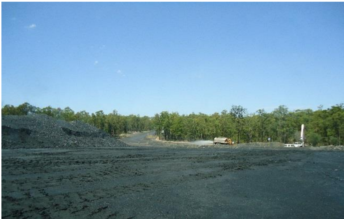
Plate 1 CHPP water cart in operation
