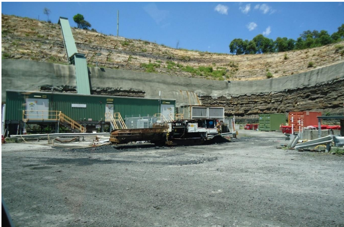
Plate 11 Abel Underground Mine Portal
