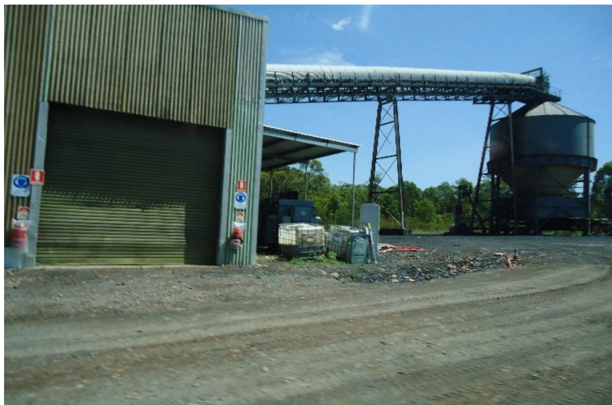
Plate 8 CHPP Areas requiring waste collection and cubes not banded
