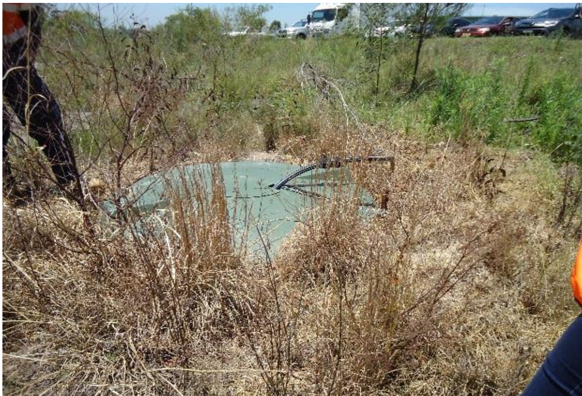
Plate 19 Redundant wastewater treatment tank
