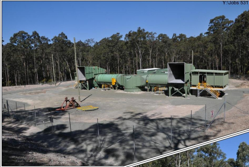
Plate 2: New Shelter Above Downcast Shaft (Date of Photography 5 September 2012) (Ref: E737E/047)
