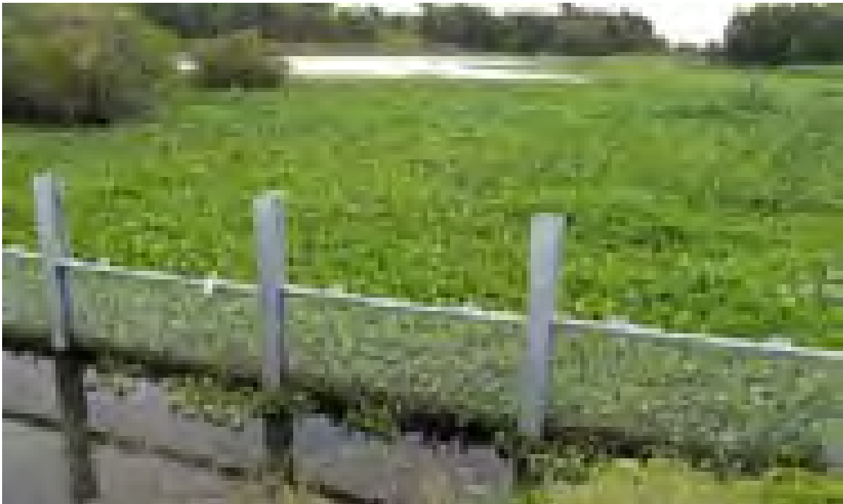
Plate 8: Water Hyacinth at the Northern Swamp inlet in 2009 showing the installation of a grate
