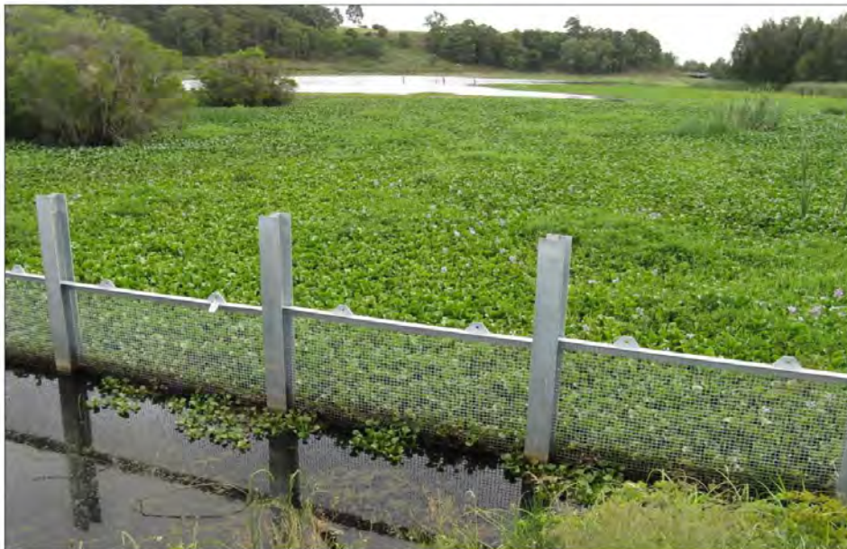
Plate 7: Water Hyacinth at the Northern Swamp inlet in 2009 (shows grate construction).
