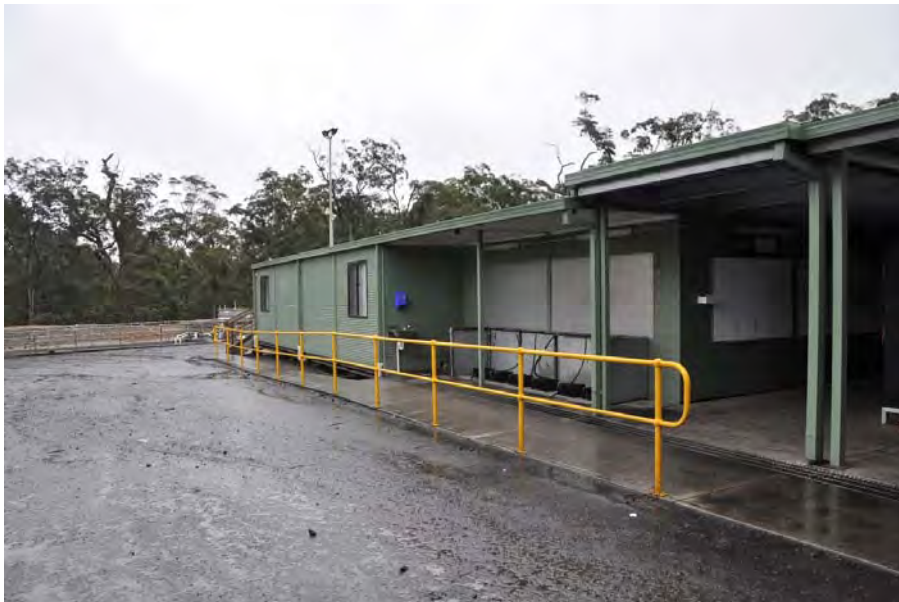
Plate 2 New Safety & Training and Administration Building (Date of Photography 10 August 2010)
