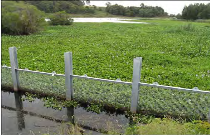
Plate 2: Water Hyacinth at the Northern Swamp inlet in 2009 (shows grate construction).
