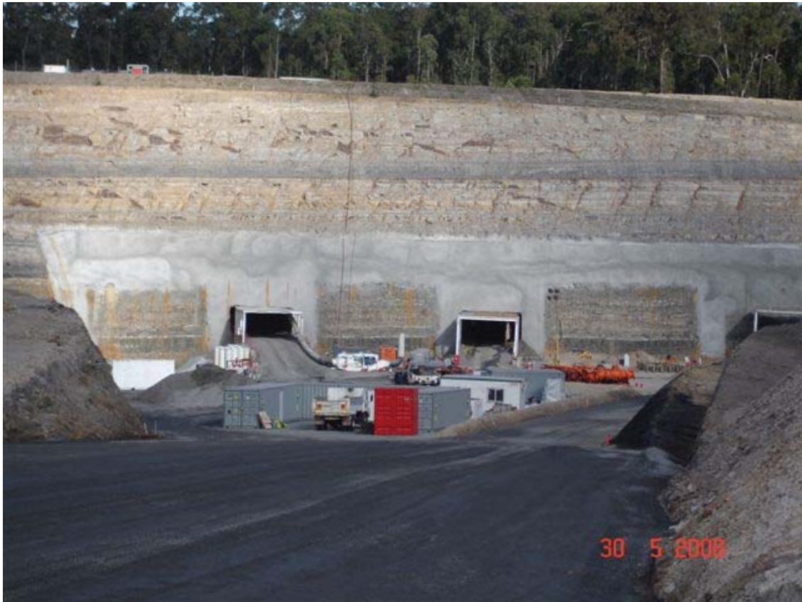
Plate 1 Mine Portals (Ref: DSC01191)
