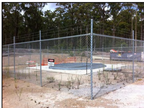
Plate 1: Existing Downcast Ventilation Shaft at the Abel Underground Mine
