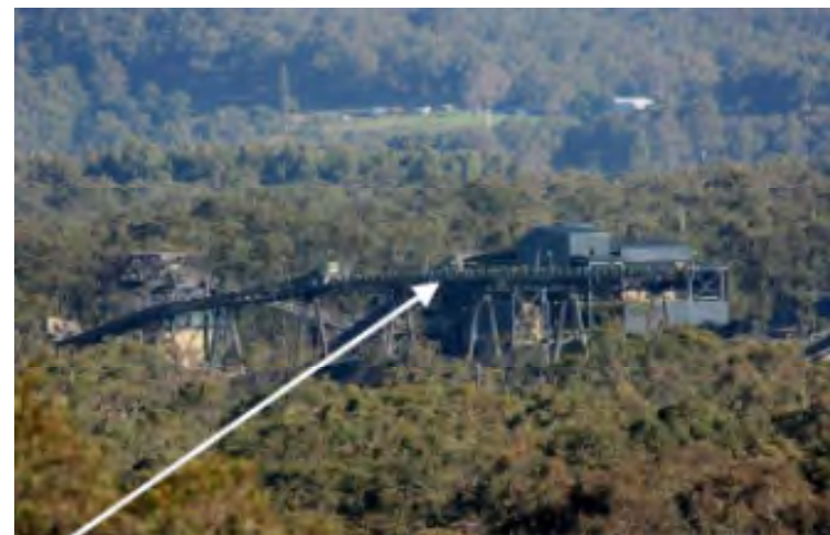
Partial enclosure of drives and conveyors of the Bloomfield CHPP for noise mitigation.
