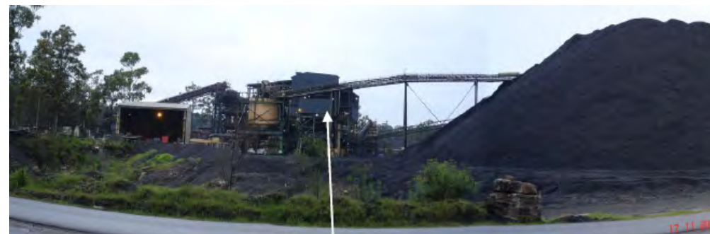
Bloomfield CHPP with new shielding on the plant to reduce noise emissions
