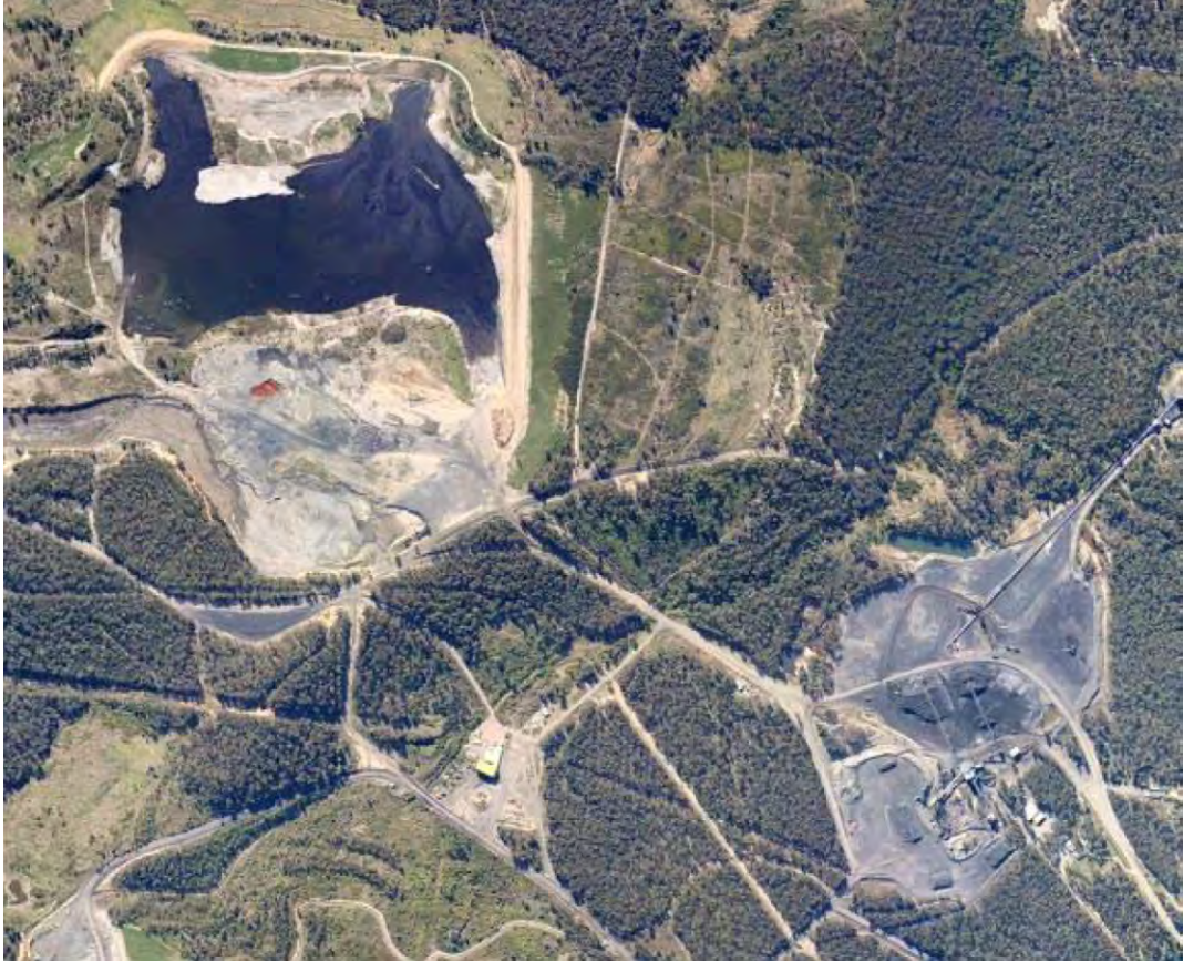
Figure 1: Aerial Photograph Showing the Bloomfield CHPP and Tailings Dam
