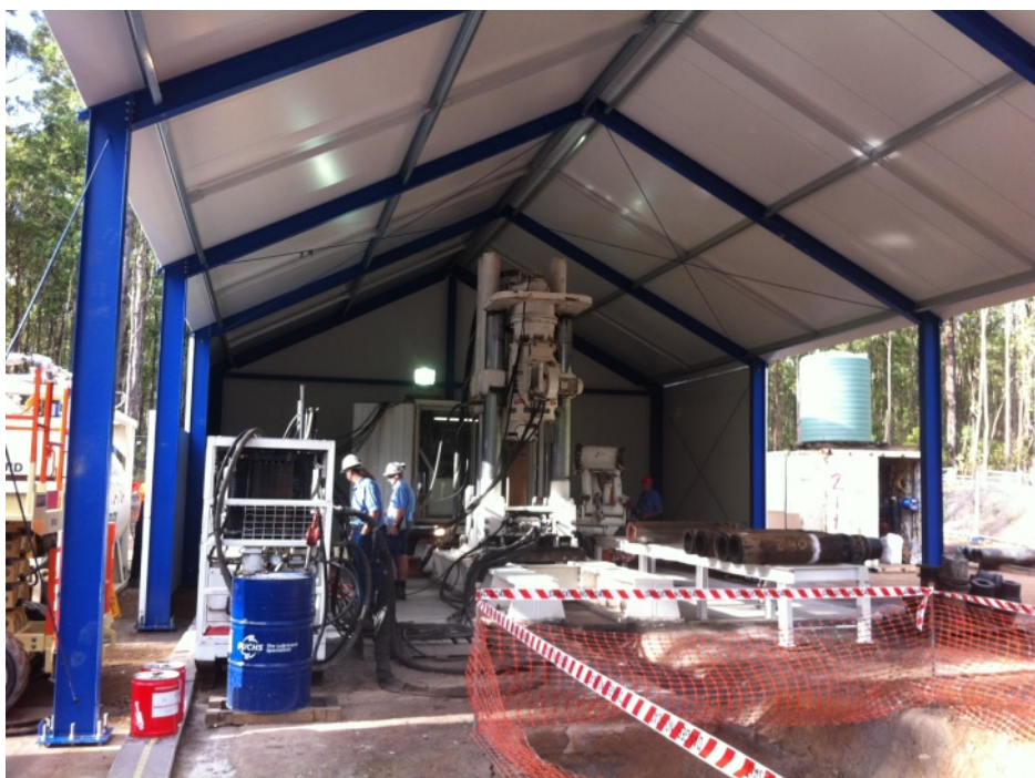
Plate 2 Abel Downcast Ventilation Shaft Construction Site
