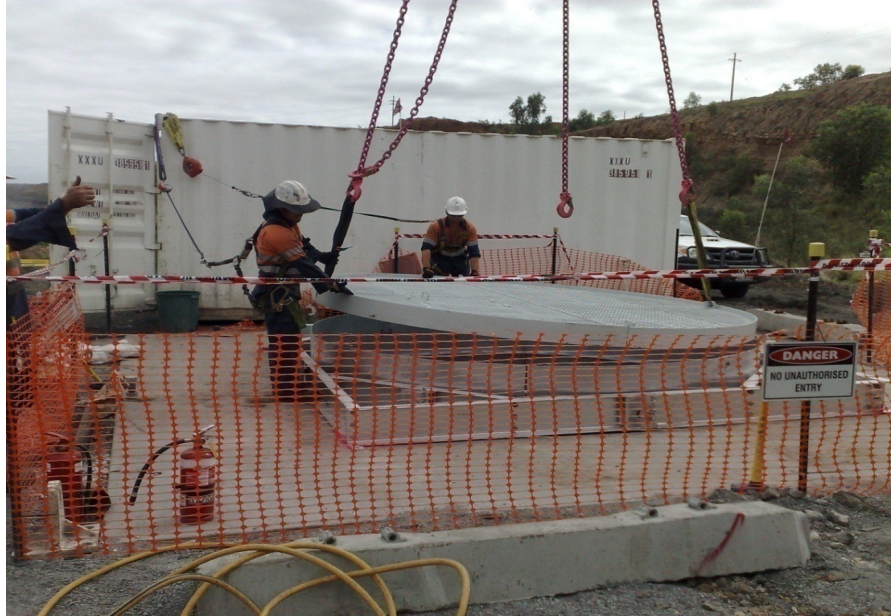
Figure 3 Photograph of typical downcast ventilation shaft construction site
