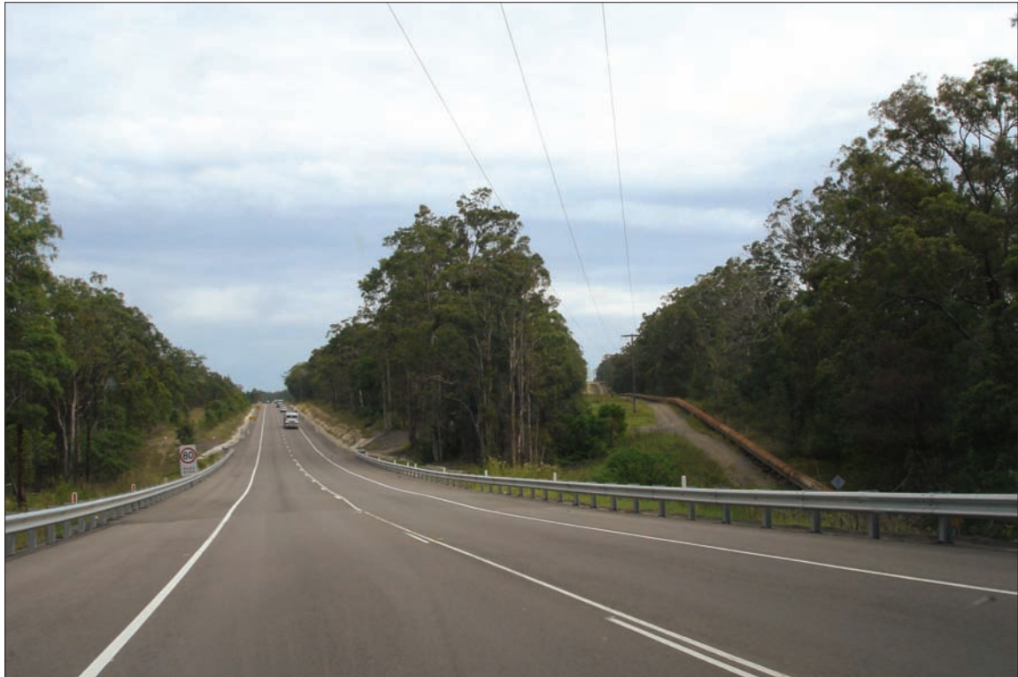
Illustration 03: The Hunter Water Corporation pipeline adjacent to John Renshaw Drive
