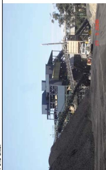
**Plate A1: Partial enclosure of the Bloomfield CHPP for noise mitigation on the northern side of the plant facing the closest residential areas.**
